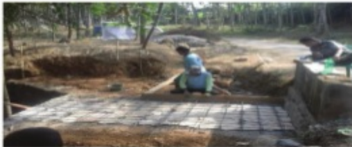
Jembatan RT. 02 – On Proses
